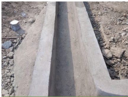
Concrete waste reused to create drains
