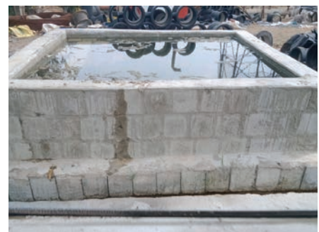
Concrete waste reused for water storage tank
